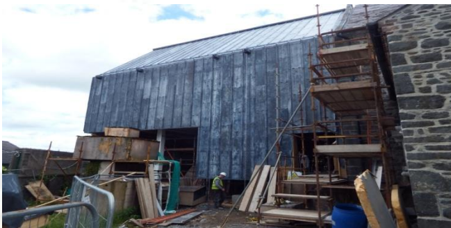
Kilkenny Room, northern elevation with scaffold removed
