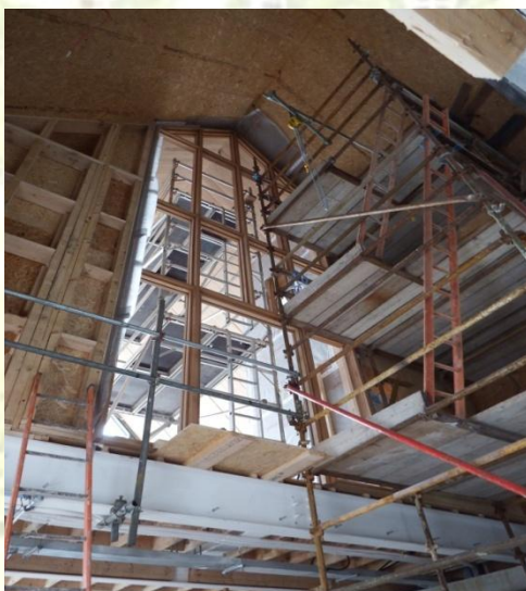
Timber screen at entrance to Kilkenny Room from Lobby.
