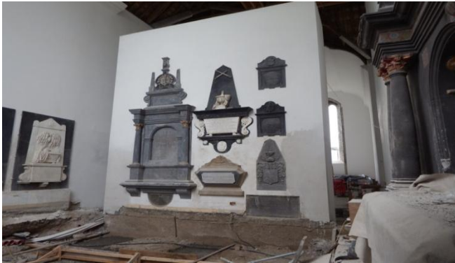
Monument wall painted and scaffold removed
