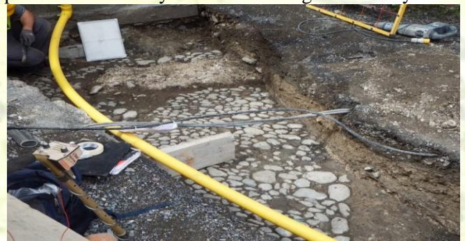
Medieval cobbled surface, indicating pathway.
