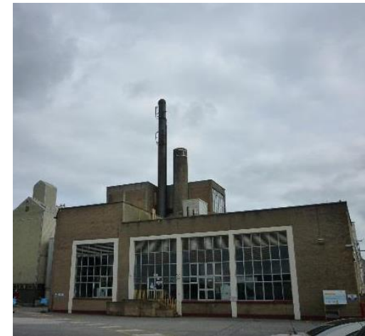
Existing – The Brewhouse
