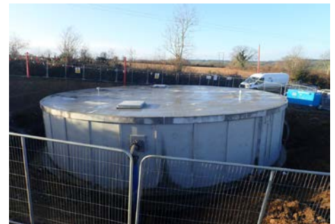
Roof installed on the reservoir at Kilmacshane, Inistioge
