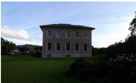
Kilrush House – Removal of defective plaster and replacement with appropriate lime plaster
