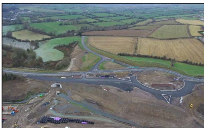
Works at Glenmore Roundabout and road underpass
