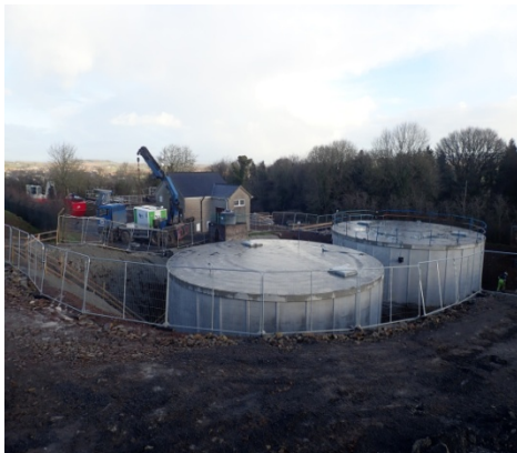
Two new Reservoirs at Grennan Water Treatment plant
