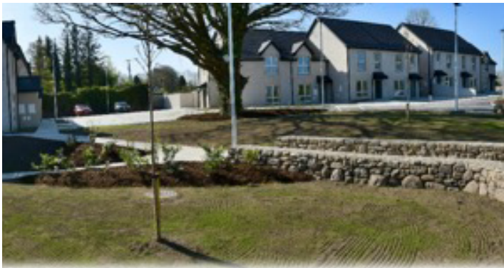
Blackwater Grove, Lower Kilmacow, Co. Kilkenny. 16 units completed April 2021 – KCC Turnkey David Flynn Construction
