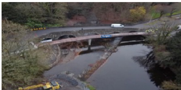
Overview with the just of the bridge Footbridge in position
