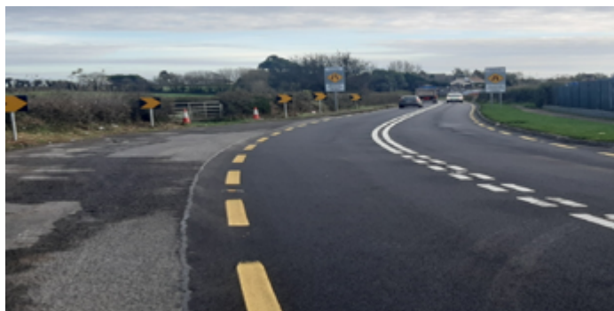
N24 West of Mooncoin. Renewed pavement, markings and signage.
