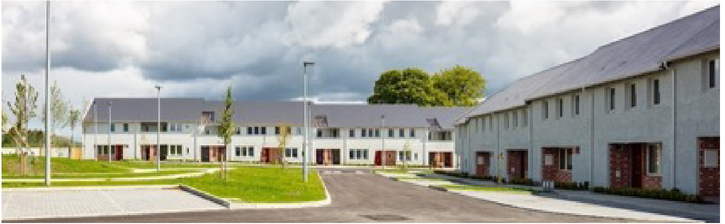
Glebeside, Donaguile, Castlecomer 33 units completed June 2021 – KCC Direct Build Designed by McGarry NiEanaigh Architects Contractor:- Cleary Doyle Construction Ltd
