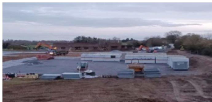
Compound setup including site storage, health and safety facilities, offices,
