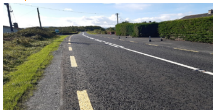
N76 Riversfield to Ahanure North – Finished Pavement
