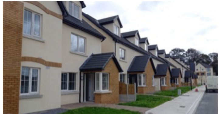
Seville Rise, Margaret's Field, Callan Road, Kilkenny City. 40 units completed January 2021 – AHB Turnkey – Respond Housing
