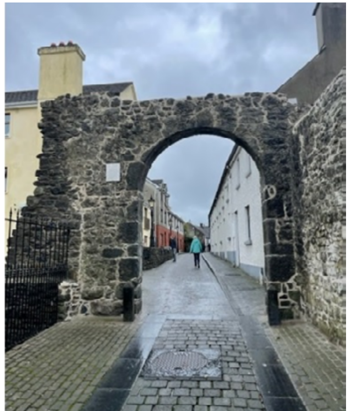
Black Friars Arch after repair and conservation works completed
