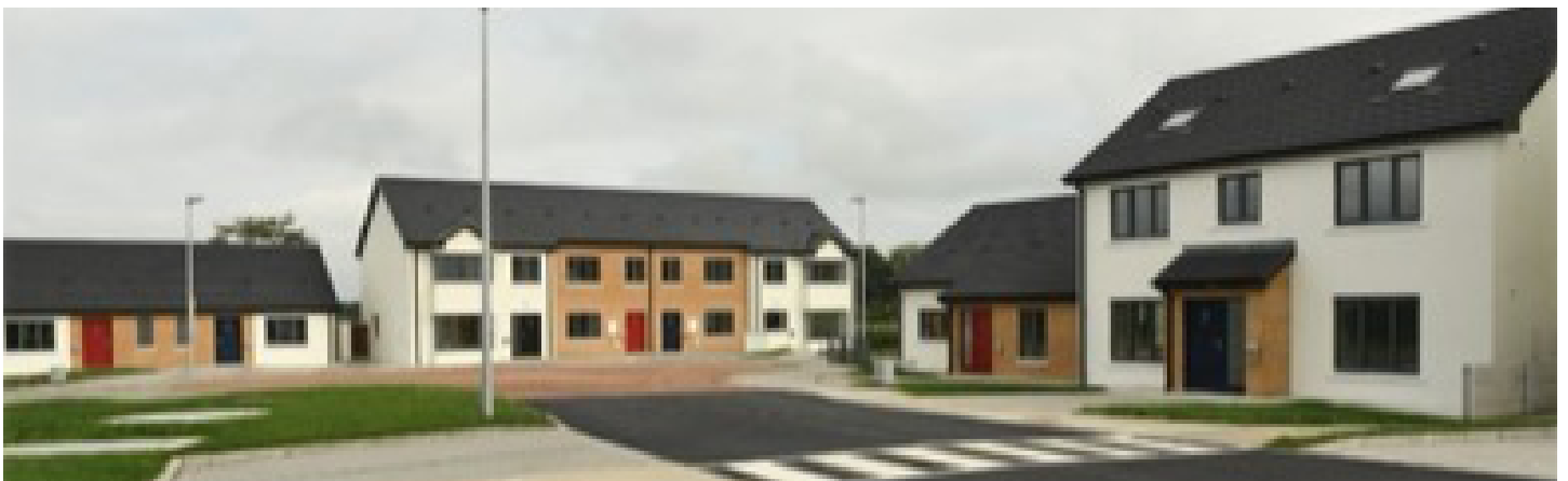
Station Avenue Phase 2, Ballyragget, Co Kilkenny. 22 units completed June 2021 – KCC Direct Build. Designed by CJ Falconer and Associates Contractor:- Thos. Kelly & Sons
