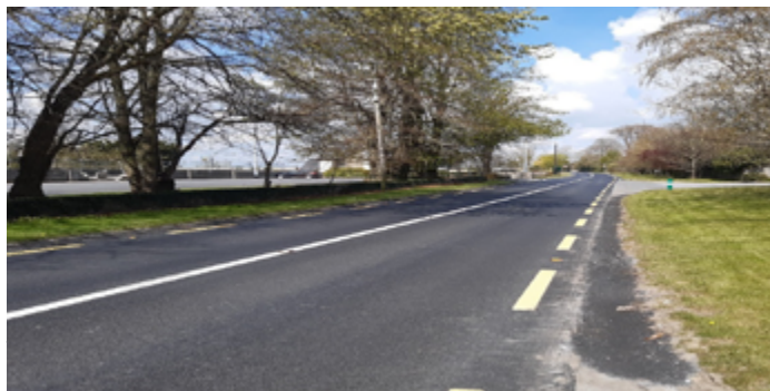
N78 Baun to Hennebrys Cross- Finished Pavement at Dunmore
