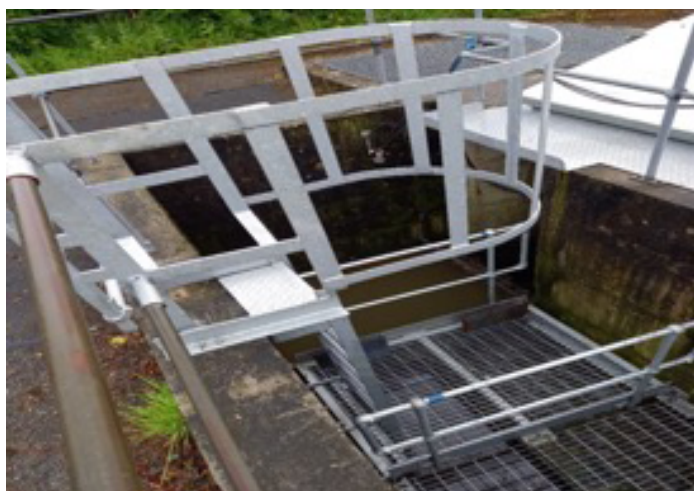
New Access Platform with Handrail support at Paulstown WWTP
