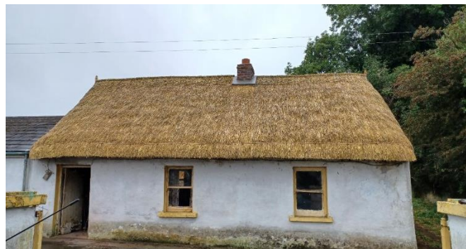
Re-roofing of Thatch Cottage, Cloneen, County Kilkenny
