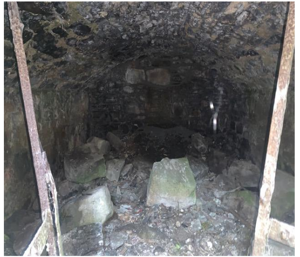
Repair of underground vault at The Thomple Historic Church & Graveyard
