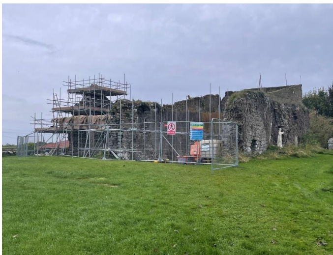
Recent photo of on going works on site at Grangefertagh
