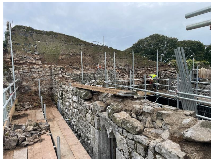
Recent photo of ongoing works on site at Grangefertagh.
