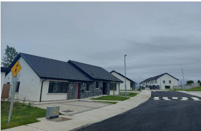
“Legan Grange and Legan Court, Thomastown – 25 units completed in September 2023”
