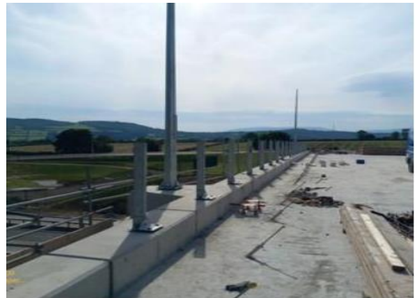
Bridge Parapet & Public Lighting Installation
