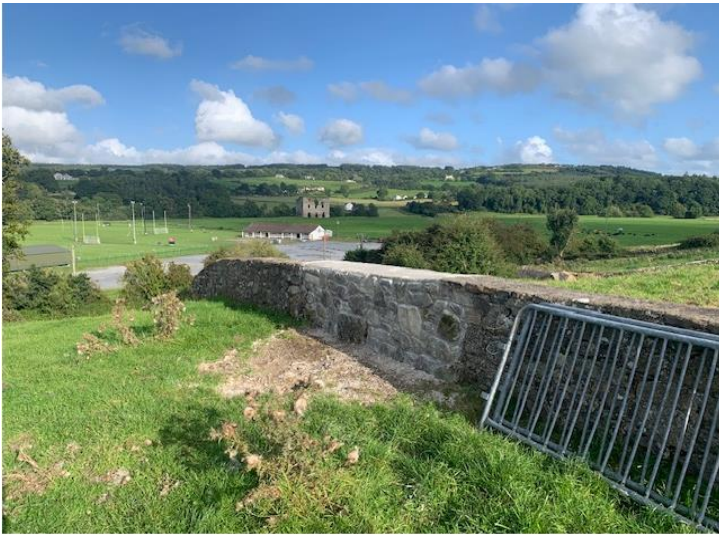
Repair of boundary wall at The Thomple Historic Church & Graveyard
