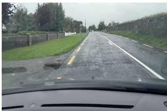
New pavement on N77 near Clintstown
